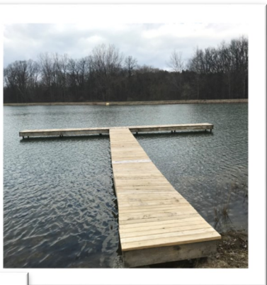
Decking for Wyandot Swimming Dock
