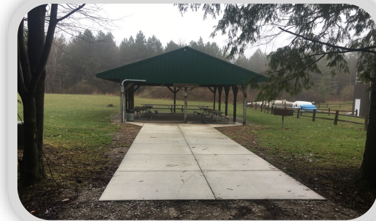
ADA Compliant Ramp for Stewards Shelter
